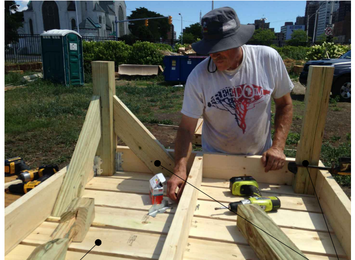
#3 Cut (4) posts to 2 feet each. Cut (8) cross braces, (4) at 2.5 feet each and (4) at 2 feet each all with 45 degree angle on each end
