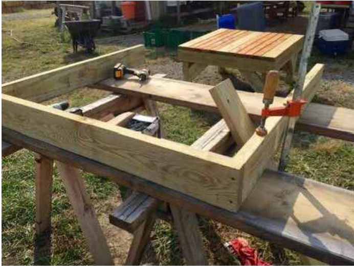
#1 Cut and assemble 4 feet by 4 feet perimeter with one joist cross member
