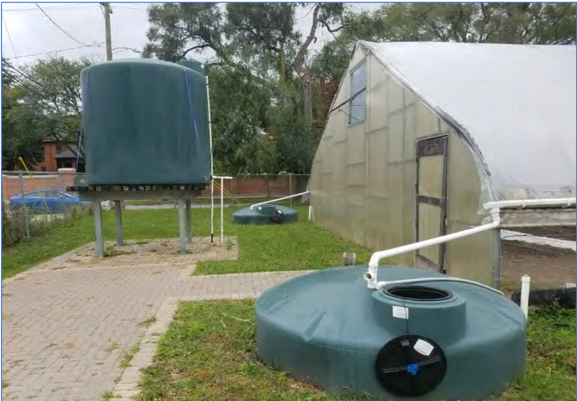
Figure 2: Two at-grade 1000 gallon cisterns and one 3000 gallon elevated cistern.
