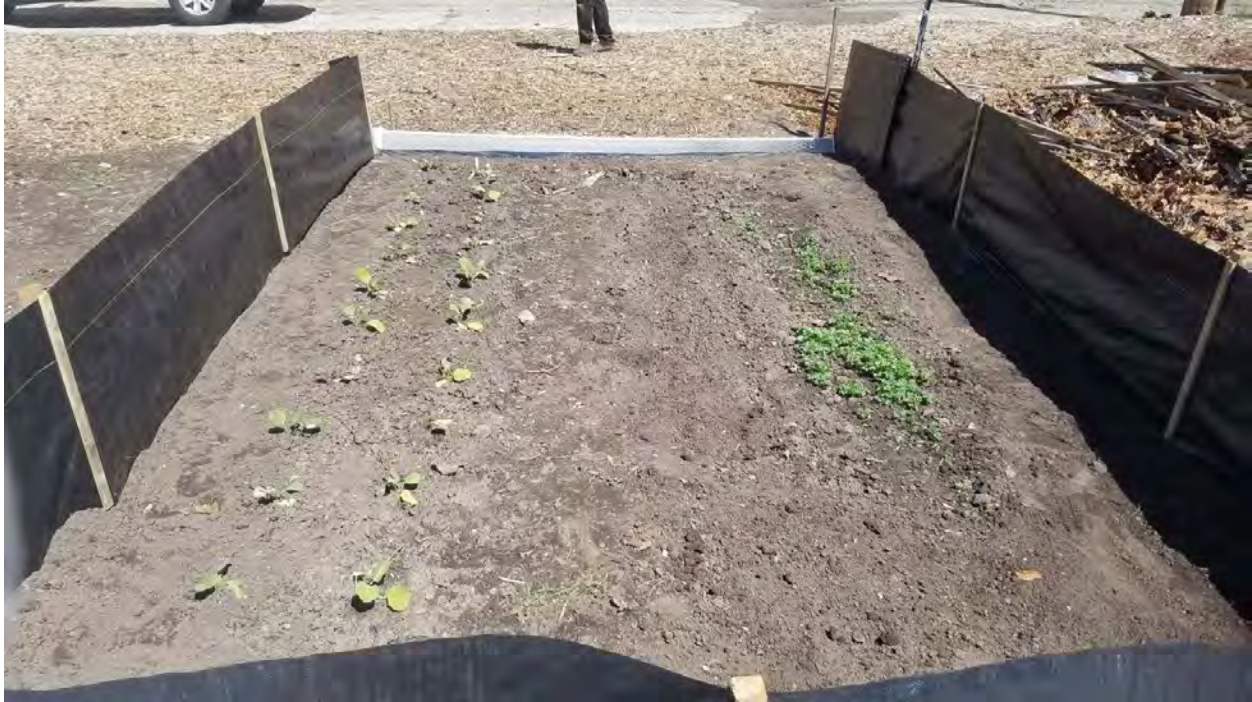
Figure 7: Earthworks Planting Bed with Runoff Collection Gutter in Background.
