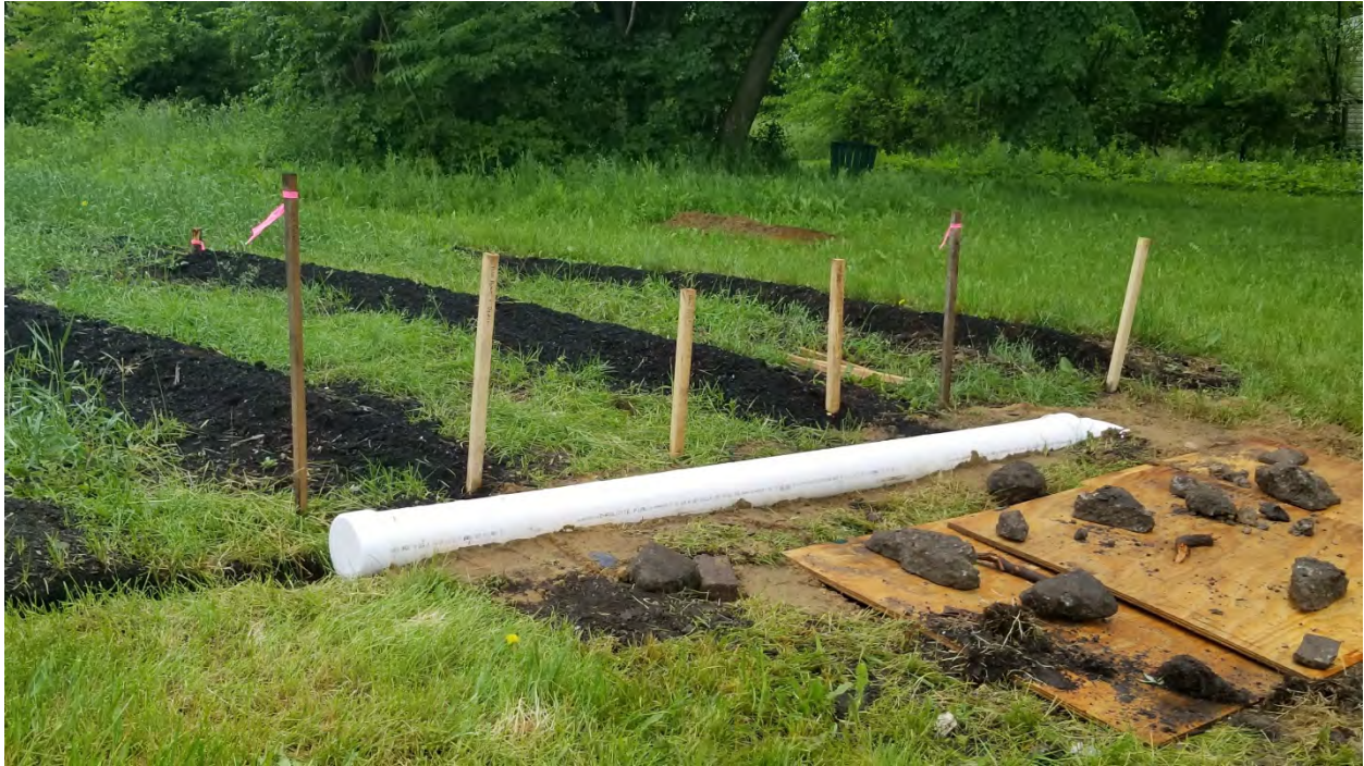
Figure 8: OAU F Planting Bed #2 During Construction
